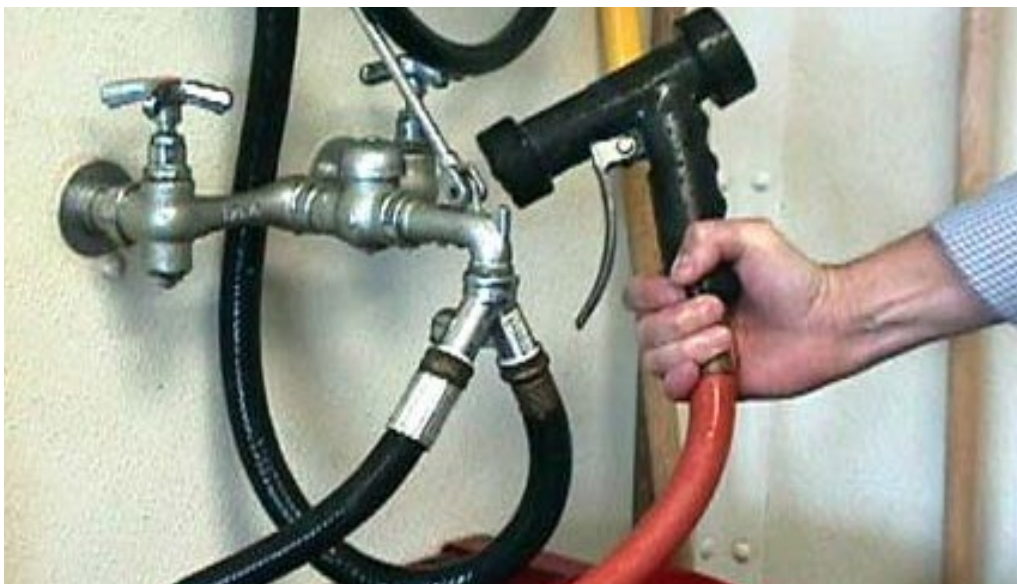
Figure 7 - Unapproved Connection
