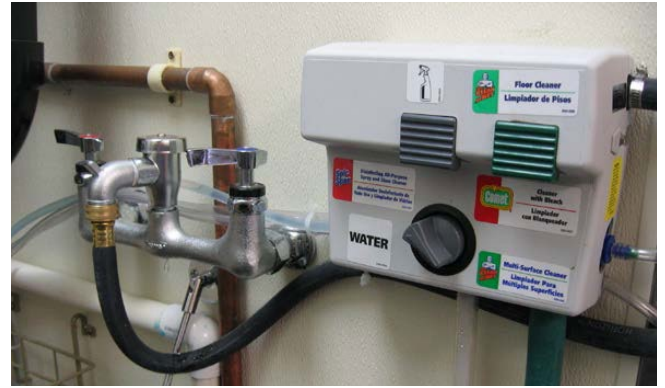
Figure 3 - Unapproved Connection
