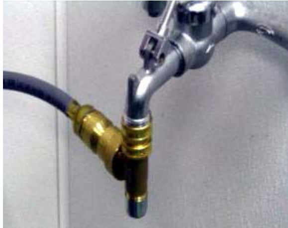
Figure 6 - Unapproved Connection
