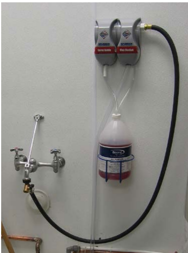
Figure 4 - Unapproved Connection
